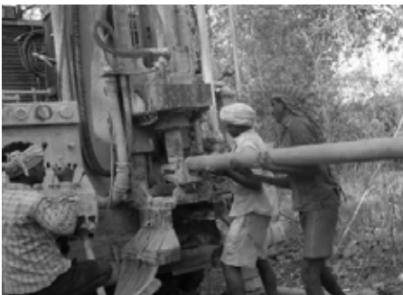
Digging was not easy but very hard labor
