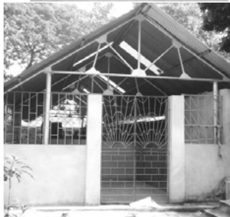
New work shed at Don Bosco
