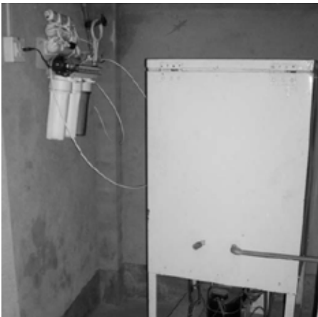
Cooling machine pump and filters
